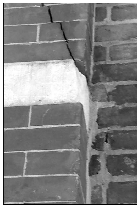
Crack in north wall to be fixed during roof repairs.
