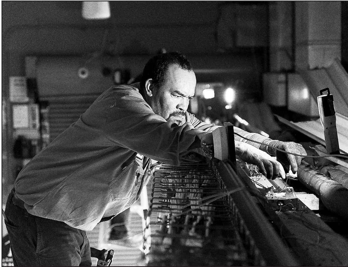
Work was done at night when the store was closed. Robert Betancour installing LED lighting above the meat case.
